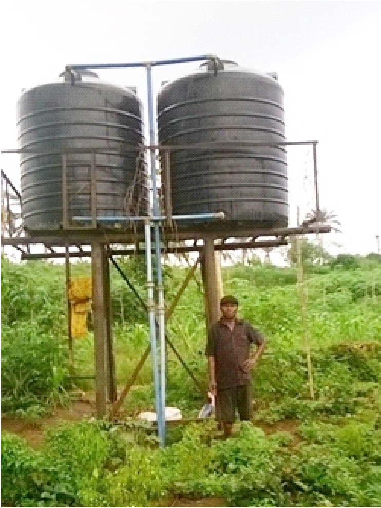
Fig 1. Small irrigation of Ata Obio Akpa, Akwa Ibom State (Photo Credit, Umoh. G.S. 2008)
